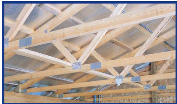
Foil insulation installed with a finishing ceiling
