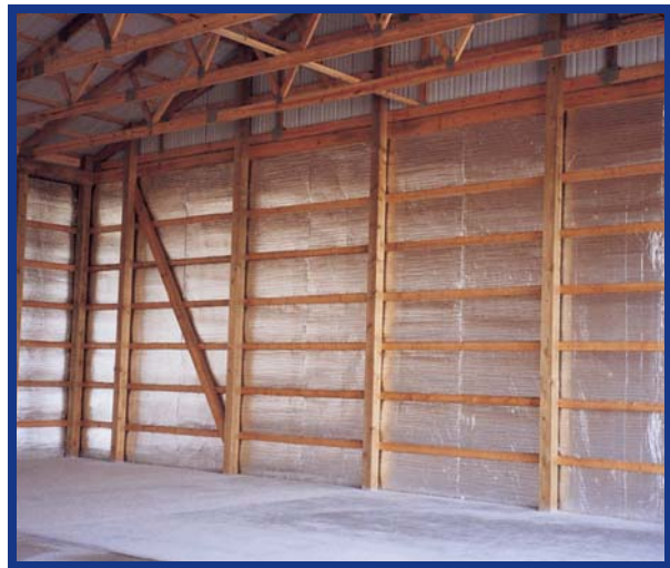
Foil insulation installed with a finishing ceiling
