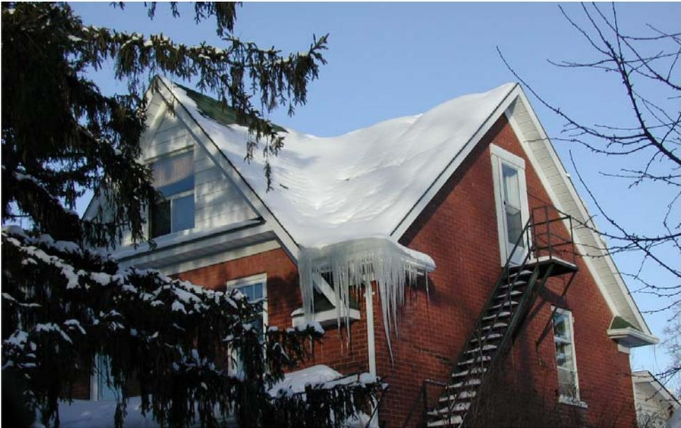
Photograph 1: An ice dam - note the snow melting on the slope above the ice dam.
